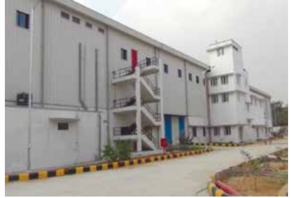
ICMF Main Hangar
