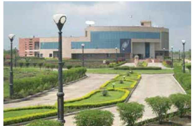
Satellite Control Centre – MCF, Bhopal
