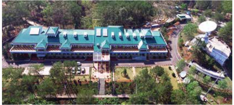
Aerial View of NE-SAC
