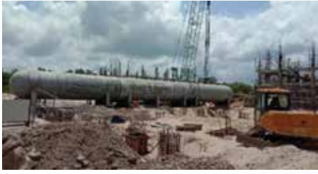
Site erection of 4.5m dia x 50m long (6 nos.) air Storage Vessel
